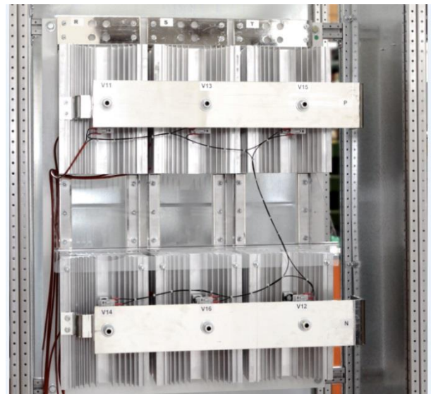
Assembling in cabinet
