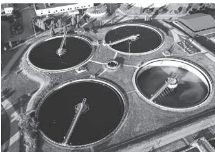
Water treatment system
